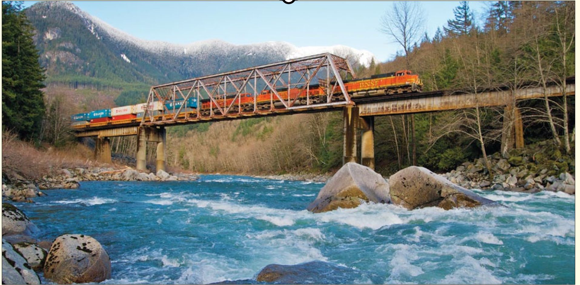
SKYKOMISH RIVER BRIDGE Approaching the long grade towards the summit of Steven's Pass, a BNSF Railway locomotive travels eastbound over the Great Northern Skykomish River Bridge near Gold Bar, Wash., on February 2, 2012. Photo courtesy: Eric Williams
